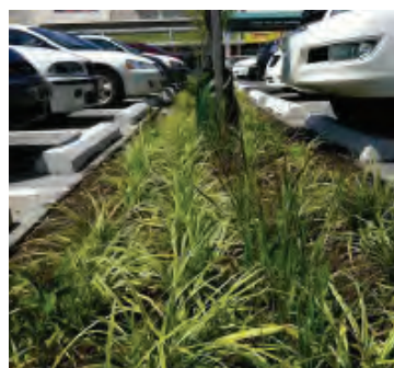
Vegetated Swale at the Trolley Station ACME in Wilmington, DE
