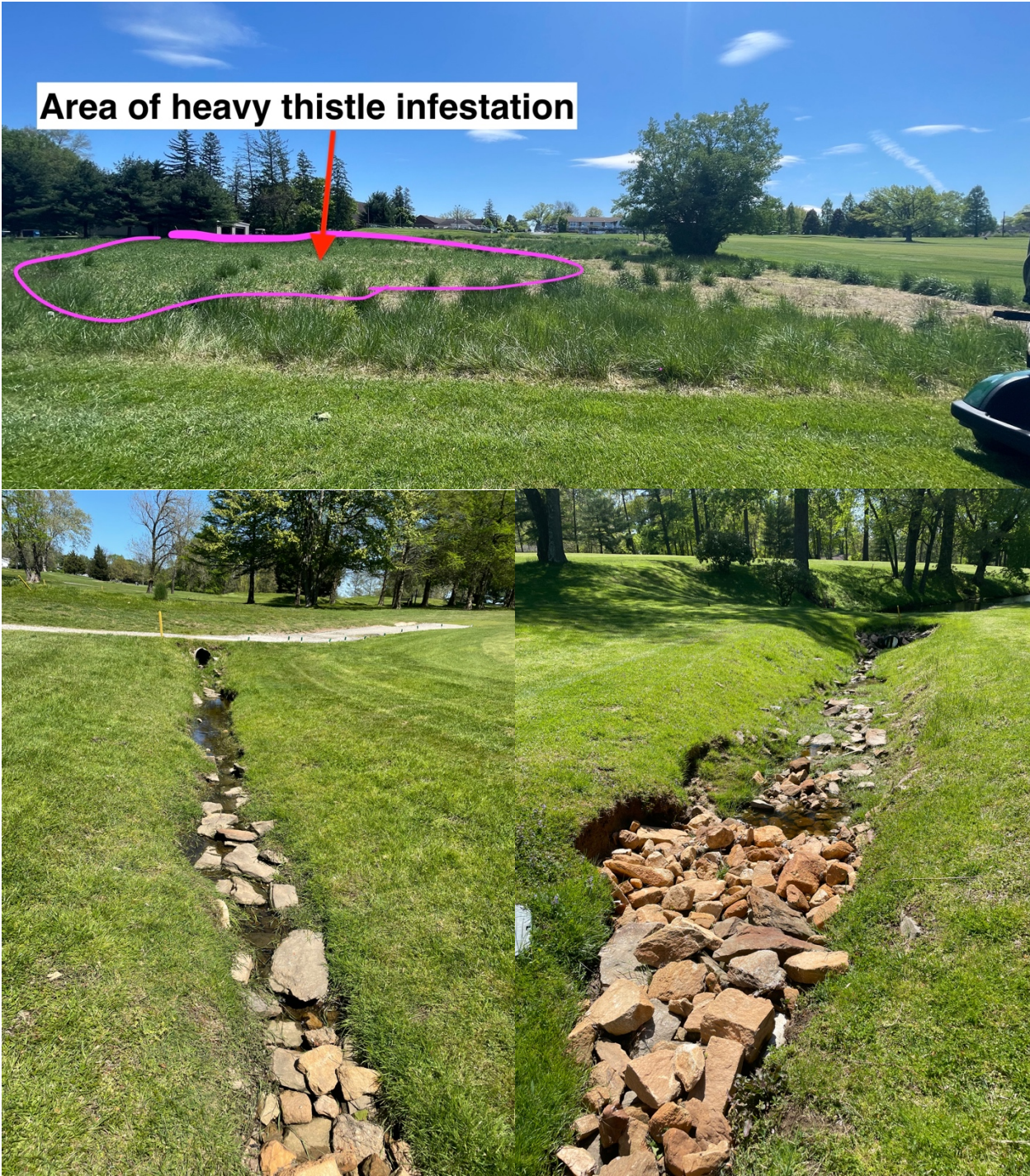
(top) existing naturalized area with Canada thistle infestation; (bottom left and right) two areas where erosive water flow has caused erosion gullies.
