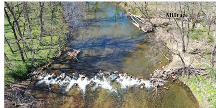
England / Red Mill (Dam #2)
