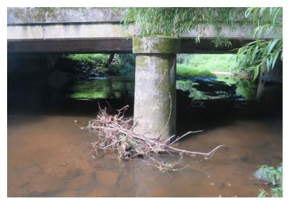
if maintenance is required. When the bridge is replaced at the end of its service lifetime, the replacement structure should be a single span bridge if feasible as that would greatly reduce the risk of blockage.
