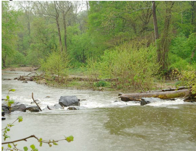
Figure 4.24. Dam No. 7, Deerfield Dam
