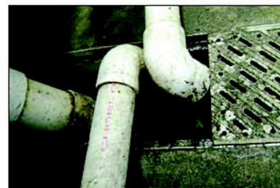
Water outflow collected and returned to the Nanticoke River
