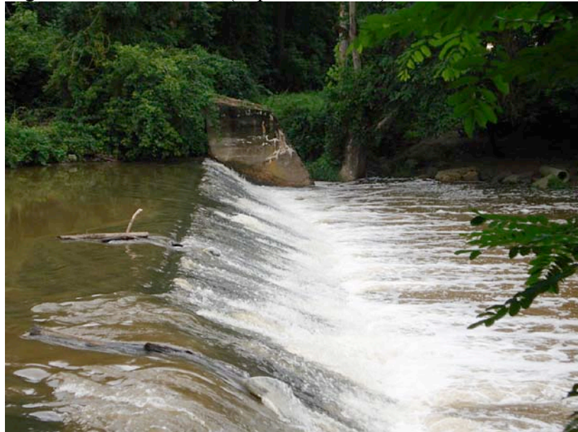
Figure 4.17. Dam No. 4 (Paper Mill Dam)
