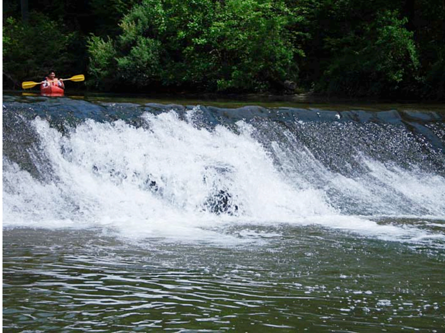
Figure 4.20. Dam No. 5 (Newark Water Supply)
