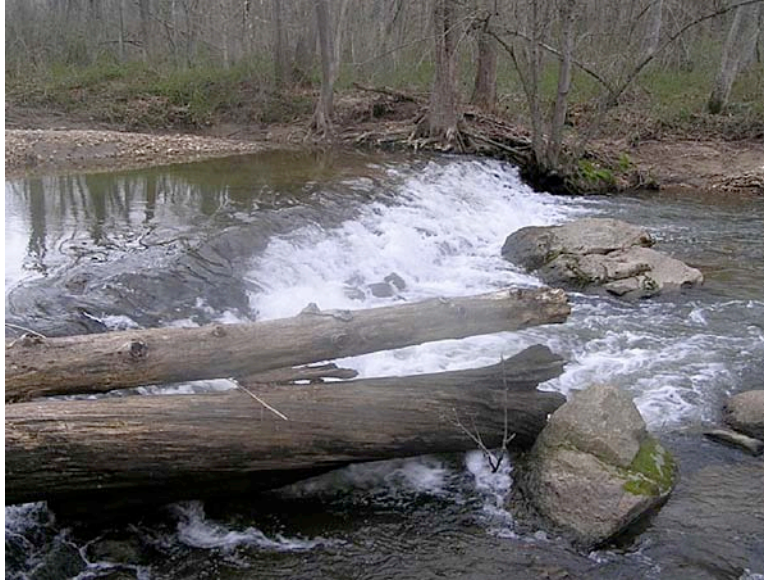
Figure 4.26. White Clay Creek Preserve Dam – Yeatman’s (or “Yetman’s”) Mill Dam
