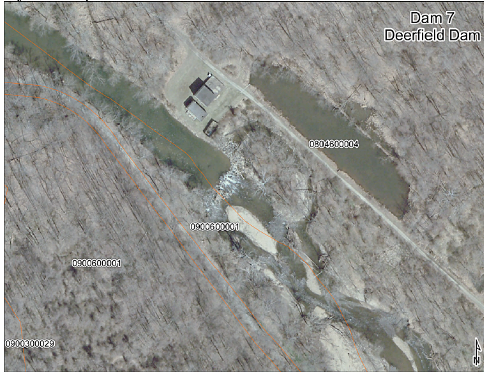
Figure 4.25 Aerial photograph of Dam No. 7 (Deerfield Dam) and adjacent tax parcels
