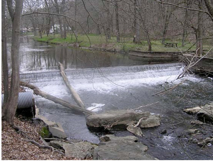
Figure 4.28. Landenberg Dam – called Thornes Factory Dam in 1847
