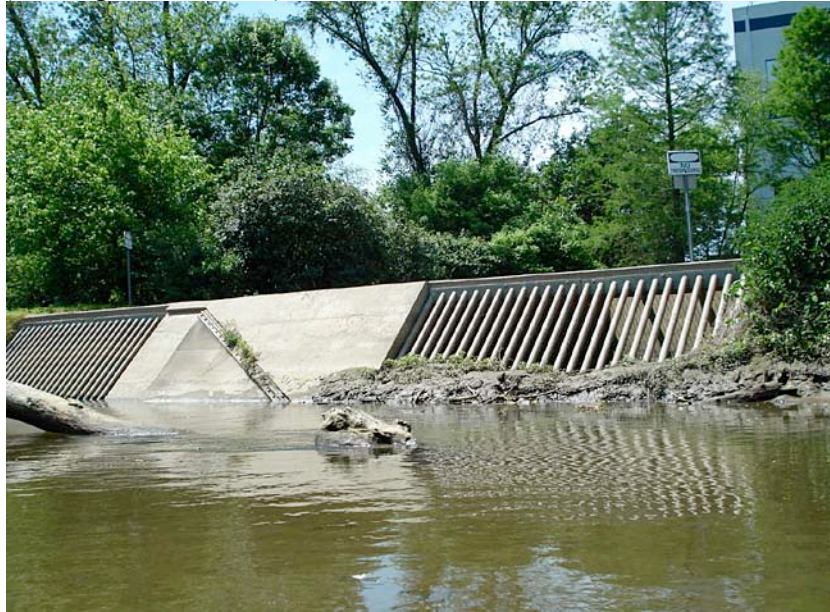
Figure 4.5. United Water Delaware's TCS (deflated) at right bank (looking downstream)
