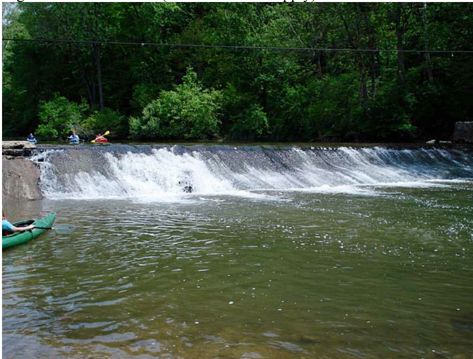
Figure 4.19. Dam No. 5 (Newark Water Supply)
