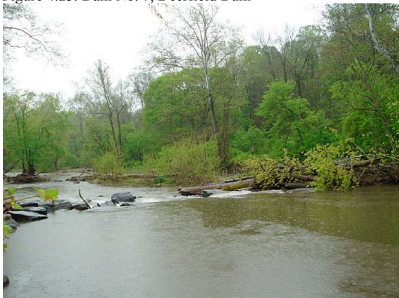
Figure 4.23. Dam No. 7, Deerfield Dam
