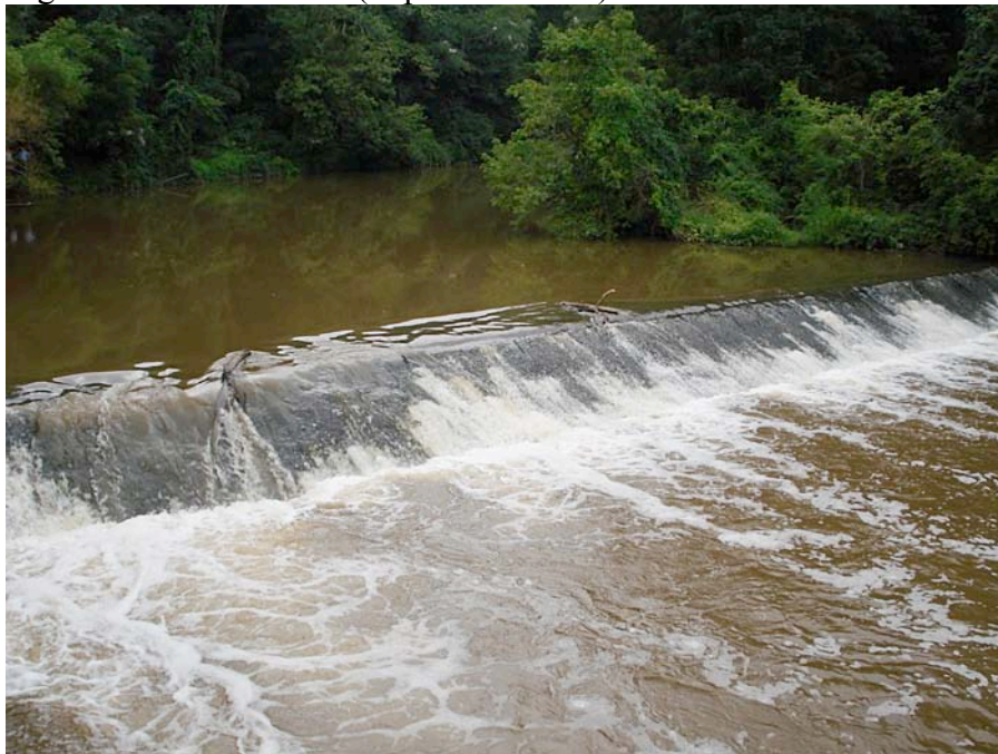
Figure 4.16. Dam No. 4 (Paper Mill Dam)
